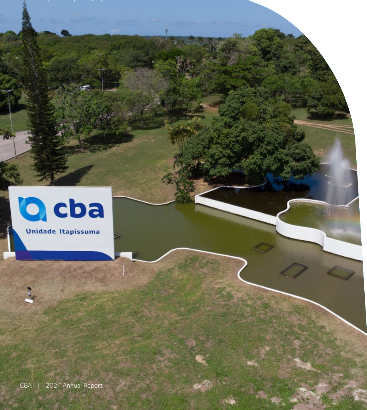
Itapissuma plant (PE)
